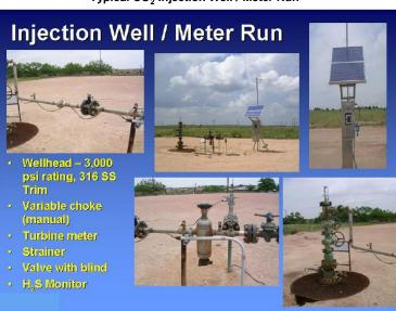
Figure 4 Typical CO<sub>2</sub> Injection Well / Meter Run <sup>9</sup>
