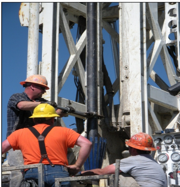
Figure C21. Photograph of securing sand basket and casing above screen.
