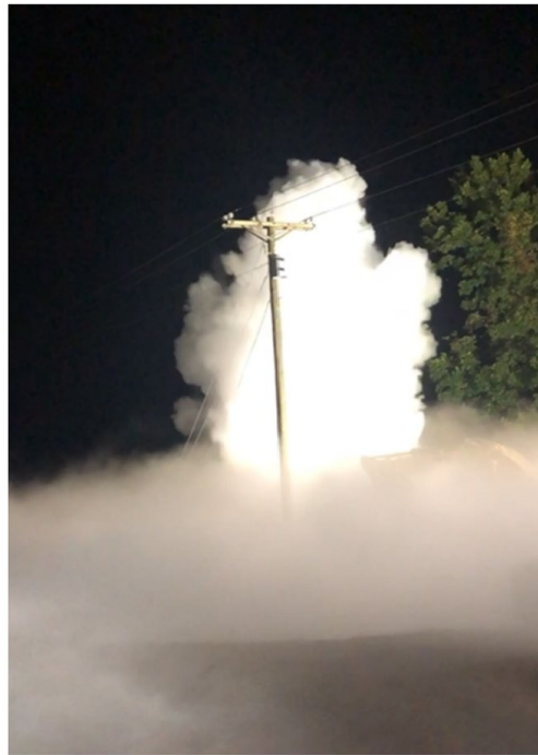
Figure 4—Night Dispersion during Blowdown Operations
