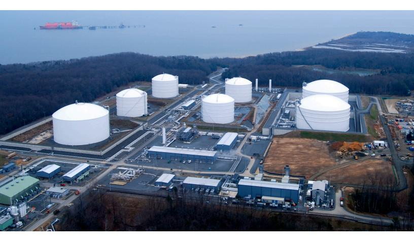
LNG, or liquefied natural gas, is a clear, odorless, noncorrosive, nontoxic liquid that is formed when natural gas is cooled to around -260 F. This shrinks the volume by about 600 times, making the resource easier to store and transport through marine shipments. LNG is not stored under pressure and is not explosive or flammable in its liquid state, and it cannot be released rapidly enough to cause overpressures associated with explosions.
