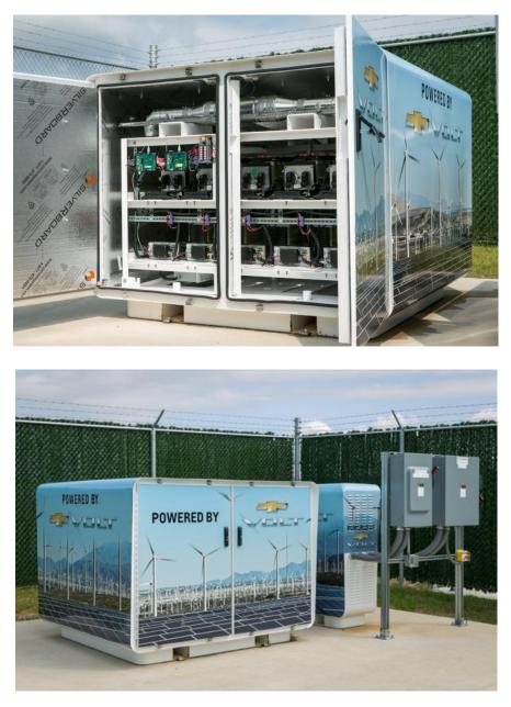
Figure 14 Energy Storage Facility Using Chevrolet Volt Batteries at GM Facility in Milford, Michigan
