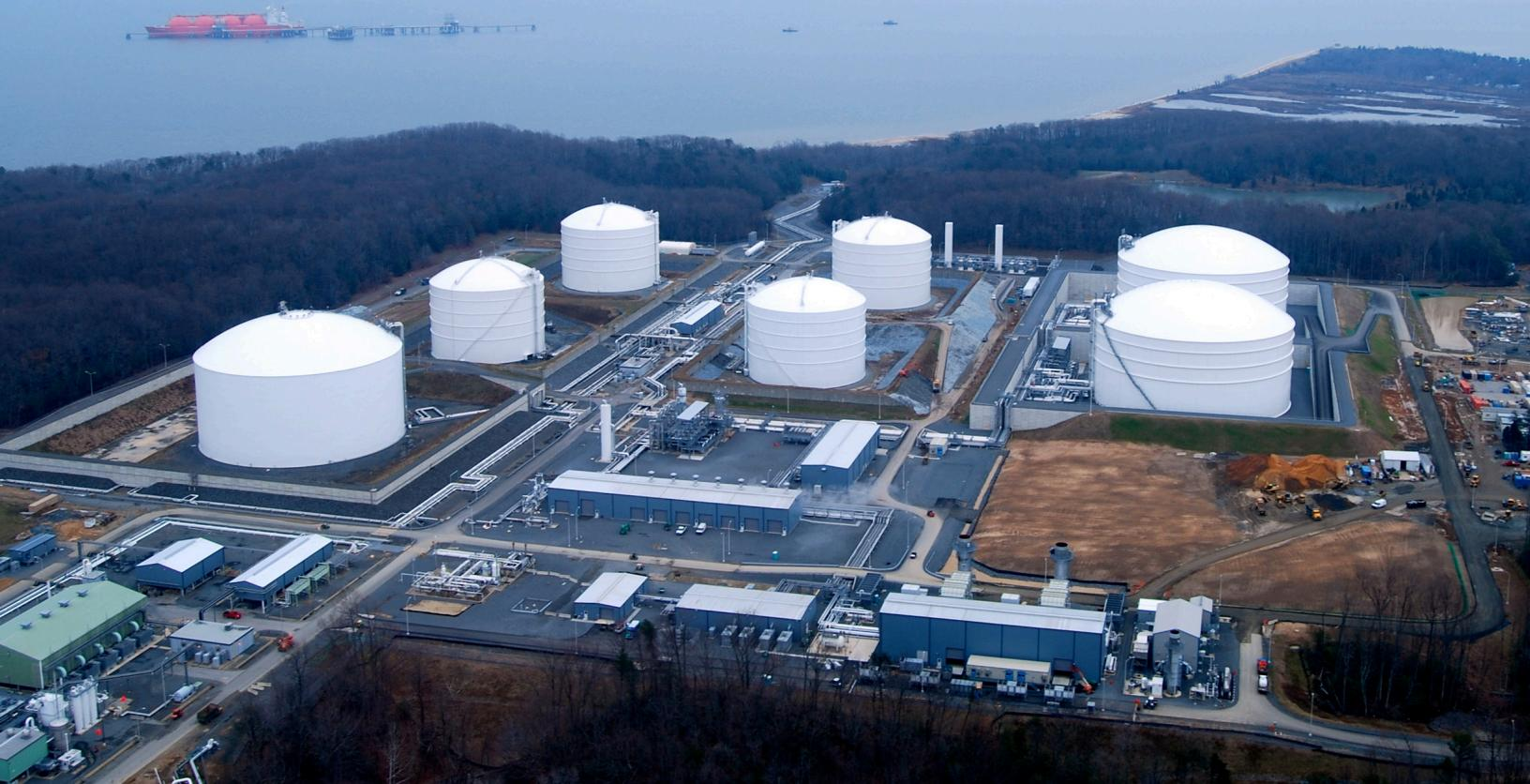
LNG, or liquefied natural gas, is a clear, odorless, noncorrosive, nontoxic liquid that is formed when natural gas is cooled to around -260 F. This shrinks the volume by about 600 times, making the resource easier to store and transport through marine shipments. LNG is not stored under pressure and is not explosive or flammable in its liquid state, and it cannot be released rapidly enough to cause overpressures associated with explosions.
